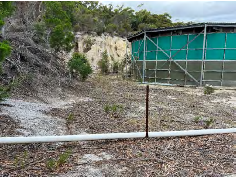
Disused Lady Barron township water holding tank near quarry
